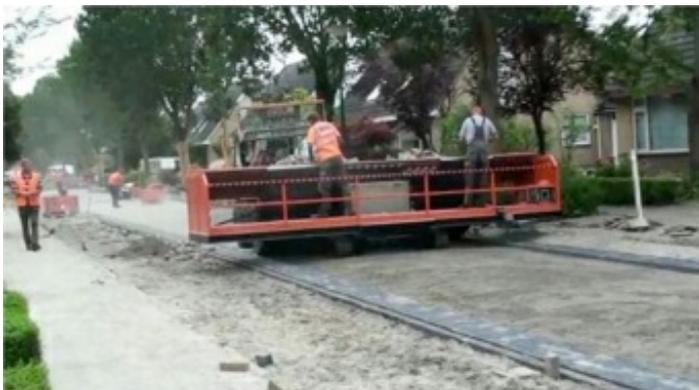
We don't have many brick-paved public roads in California, but apparently they have enough in Holland to warrant developing a brick laying paving machine. Tiger-Stone is a Dutch paver laying machine that produces brick roads. Paving bricks are dropped into the angled trough by a front-end-loader. Men help to spread them in the trough as they drop into the forming jig. As the electrically operated crawler moves forward along a pre-laid sand base layer, all the bricks are packed, held
