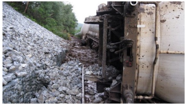
A 24-wagon freight train derailed at Tulloch on the West Highland line
