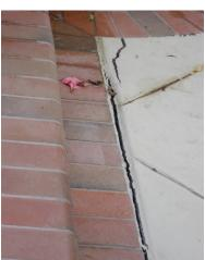
**Settlement.** As expansive soil dries out, it will shrink. If it shrinks enough, the ground surface may drop perceptably. Supported improvements may also drop or tilt and develop cracks or separations. This type of ground movement may also displace improvements laterally, resulting in cracks or gaps at joints.
