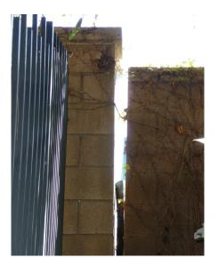
The lateral movement near the tops of slopes will often displace improvements in that area; patio slabs may develop gaps where they meet the house; columns for patio structures may develop a "lean" if the tops are attached to the home; gaps may develop around the perimeter of pools; and the construction joints in side yard walls may get wider in response to this type of ground movement.
